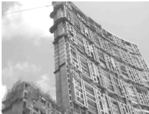
Formwork marvel at PLANET GODREJ - Byculla
