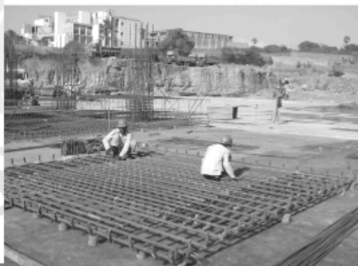
Reinforcement placing at ORCHID OZONE MALL - Dahisar
